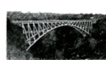
Victoria Falls Bridge, Africa. A masterpiece in steel on the Cape to Cairo Railway. The track is 420 feet above the river.
