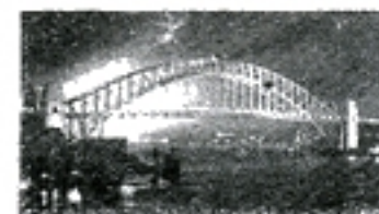
Sydney Harbour Bridge, Australia. A steel parabolic arch nearly ½ mile long. Cost of building £4,217,721/11/10.
