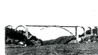
Svinesund Bridge, Norway. Steel and reinforced concrete. Main arch is a Parabola; small arches semicircles.
